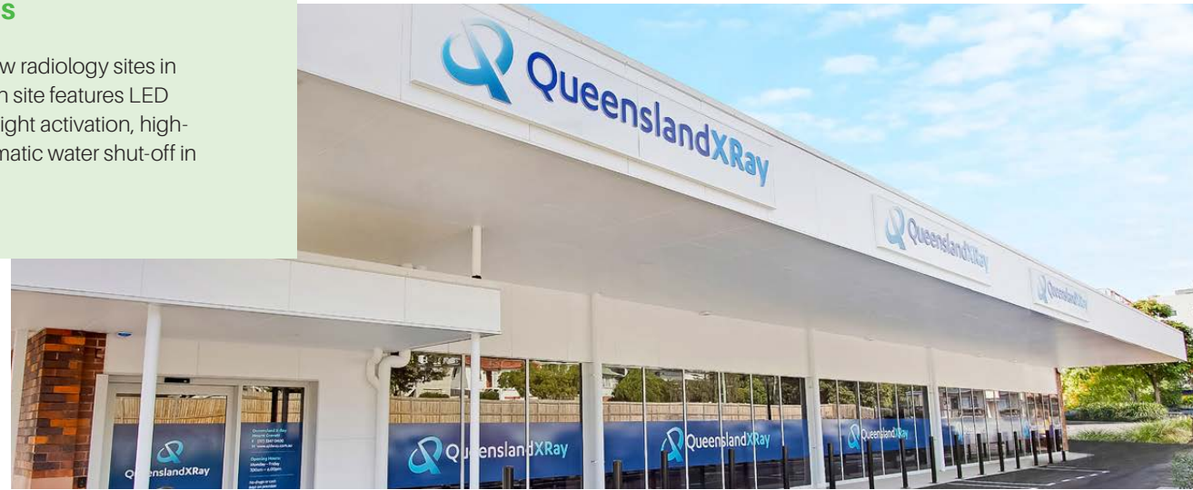
▶ New Queensland X-Ray site in Mt Gravatt, Queensland
